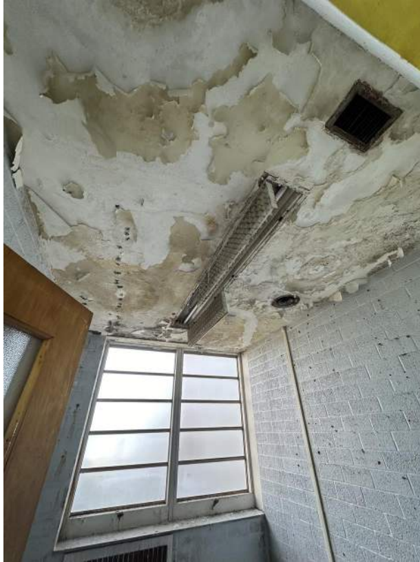
Electrical – Typ. Light Condition
