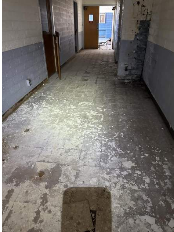
Architecture – Asbestos Floor Tile
