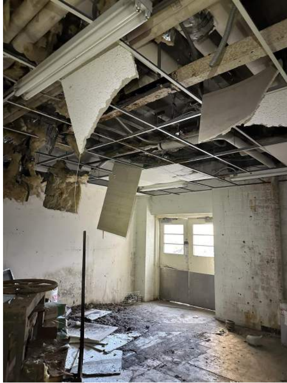
Architecture/Structural – Basement – Typical Condition
