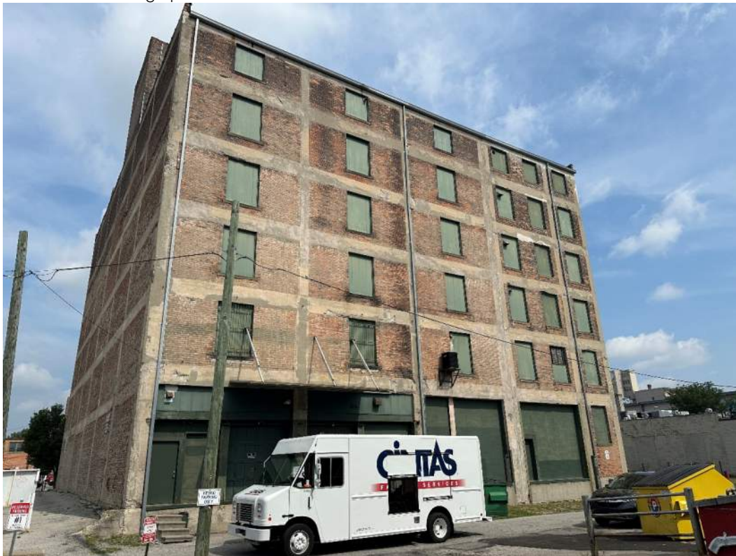
Photo 6: 2025 Photograph – back elevation. Credit: Thomas Porter Architects
