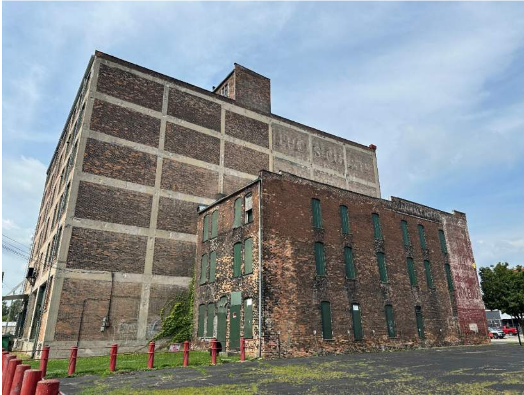
Photo 7: 2025 Photograph – northeast elevation. Credit: Thomas Porter Architects
