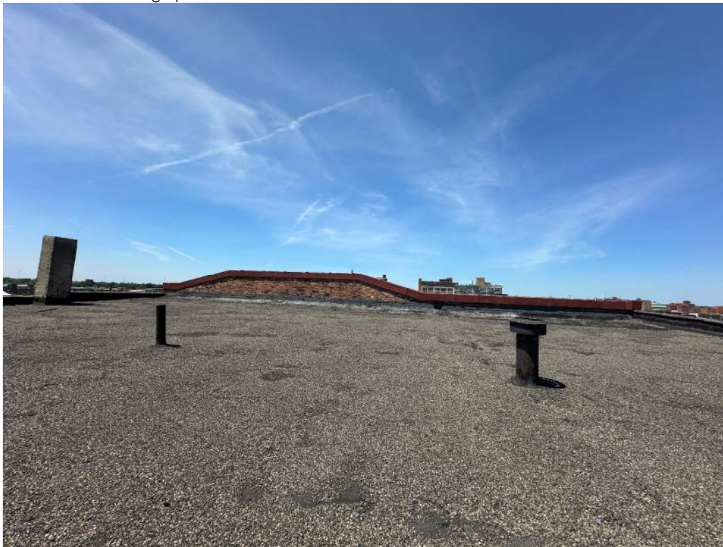
Photo 14: 2025 Photograph – roof. Credit: Thomas Porter Architects
