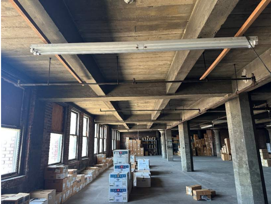
Photo 11: 2025 Photograph – fourth floor. Credit: Thomas Porter Architects
