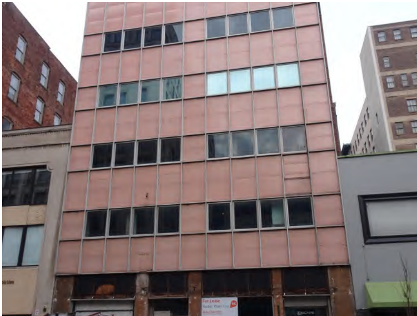
317 N SUPERIOR | INTERIOR DEMOLITION
