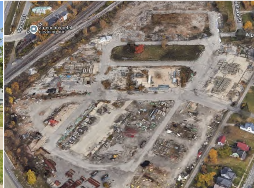
1045 POST | PORT AUTHORITY
