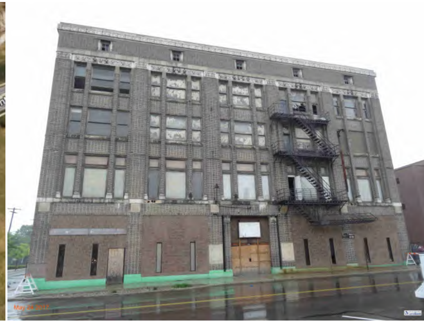
401 MAIN | INTERIOR DEMOLITION
