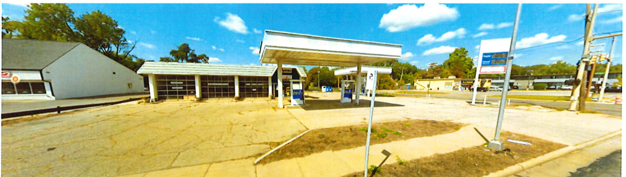
Google Street View (Sept 2025) image of the subject property from Reynolds Road.
