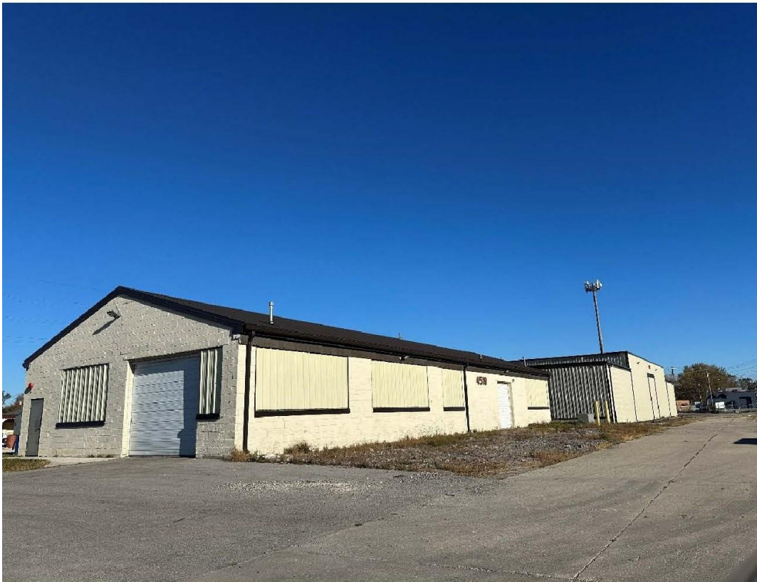
Photo 8: 2025 Photograph – outbuildings. Credit: Thomas Porter Architects
