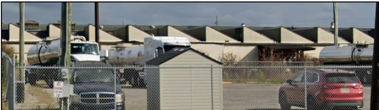
Google Street View image of the sawtooth roof line from Detroit Avenue.
