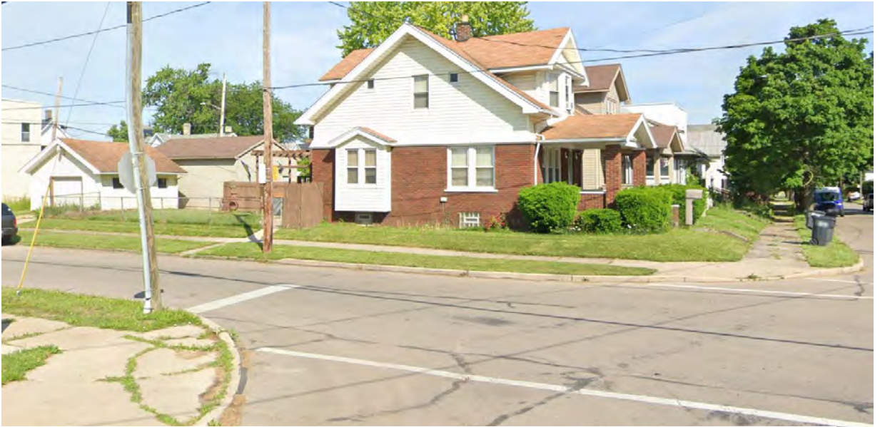
Figure 16 ADA accessible ramps are missing at the intersection of Mott Avenue and E Broadway Street
