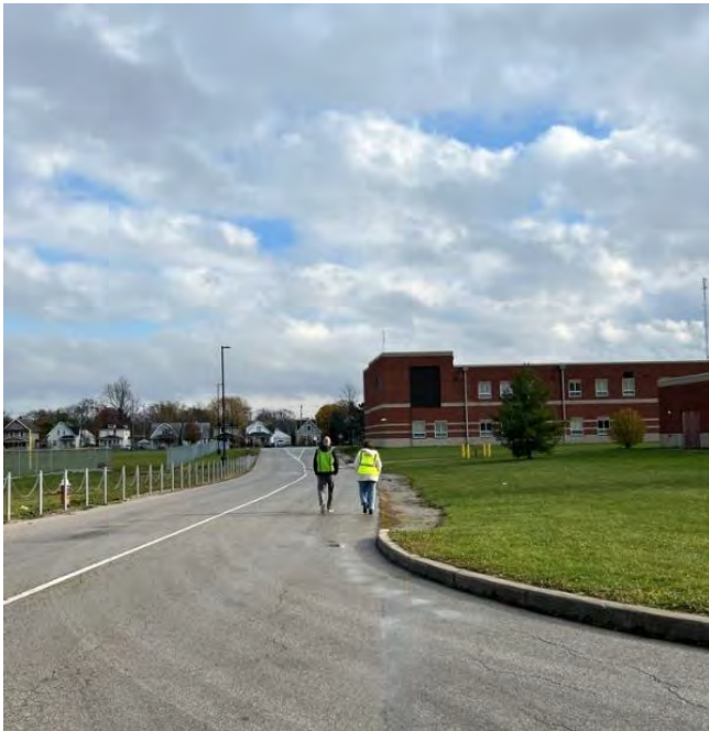
Figure 3 Missing sidewalks along the internal road around the school.
