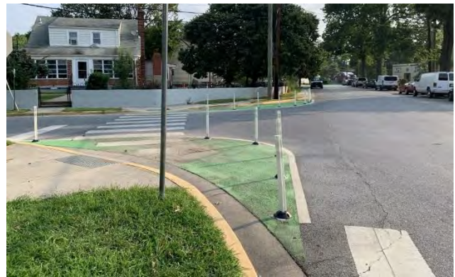
Figure 28 A project in Hyattsville, Maryland uses paint and flexible delineator posts as an interim measure to reduce the curb radii at an intersection. This strategy encourages drivers to slow down while turning
