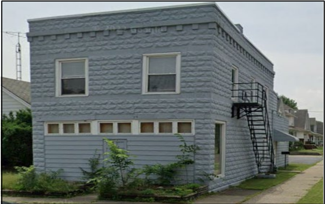
Google street view image of the subject property from Kelsey Avenue (June 2022).
