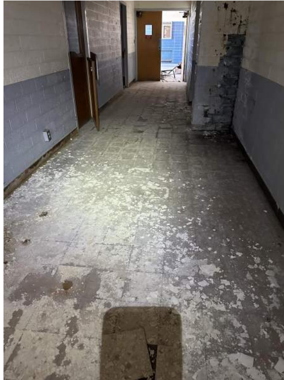
Architecture – Asbestos Floor Tile
