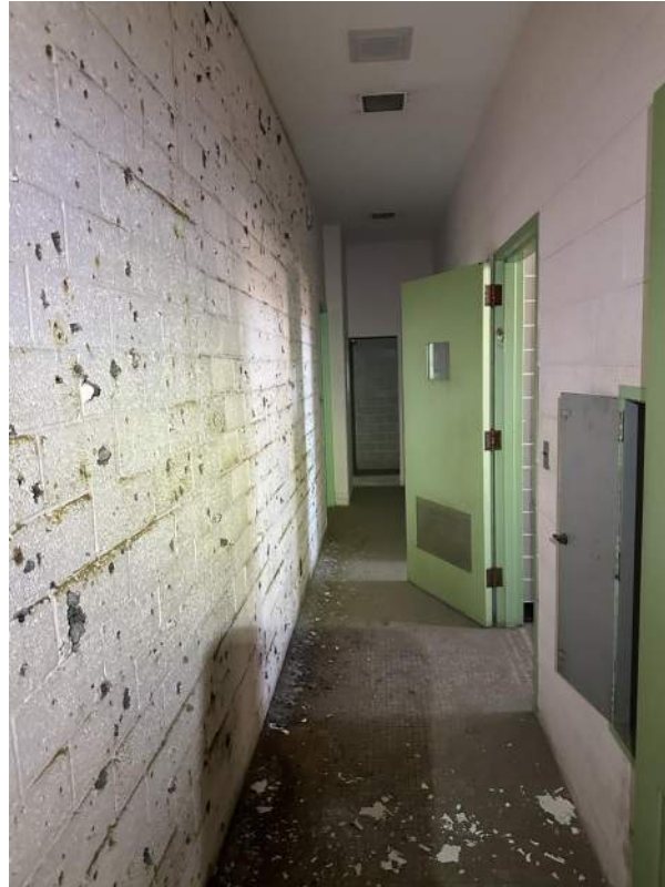
Architecture/Structural – Typ. Interior Block Moisture Blow-outs
