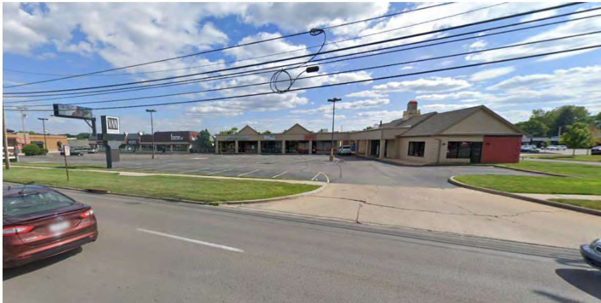
Google Street view image of existing shopping plaza to be demolished.
