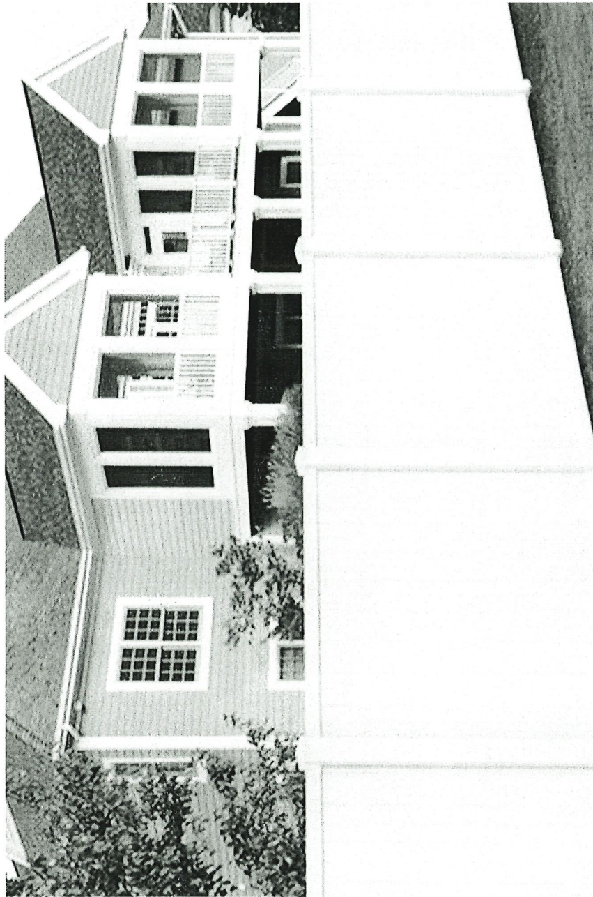
6' high white Belmont fence — shows fencing type to be used
