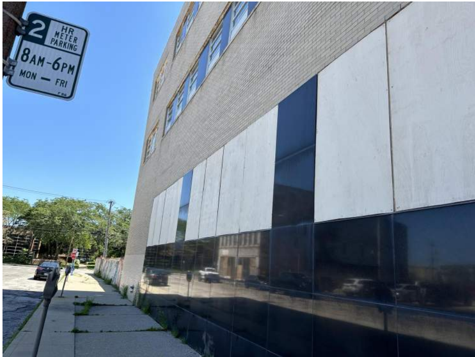
Architecture/Structural – Northwest Facade
