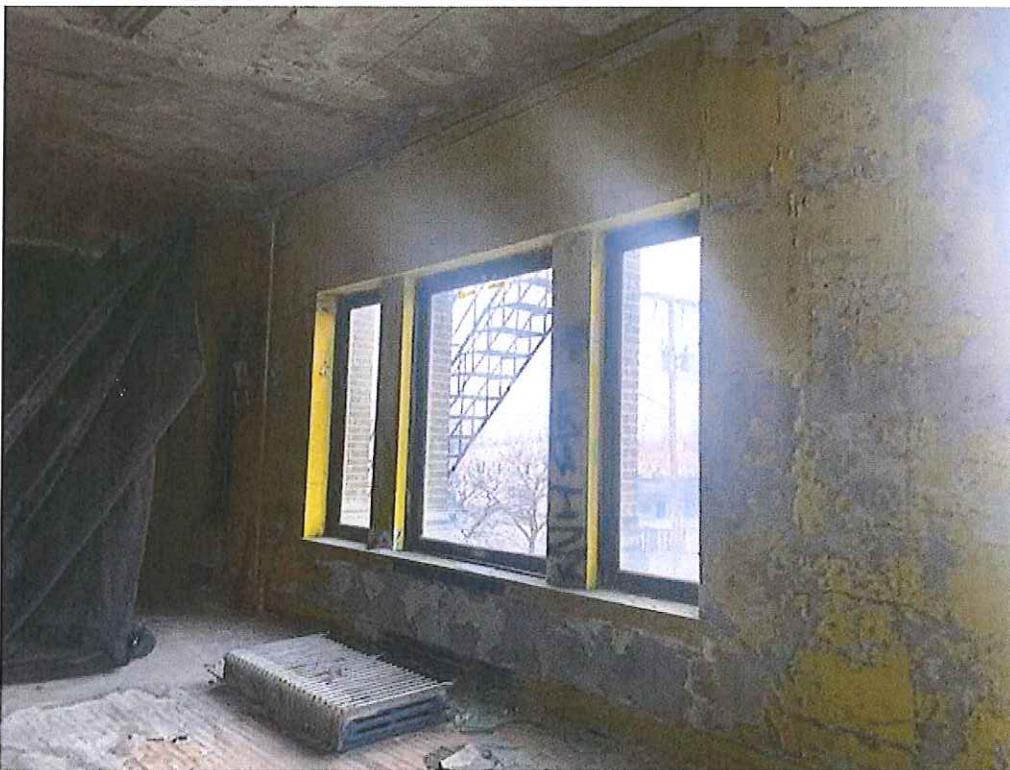
Photo 7: 401 S. Main St. circa 2020. Interior wall & window. Credit: ARK Development
