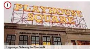
1 Lagrange Gateway to Riverwalk
