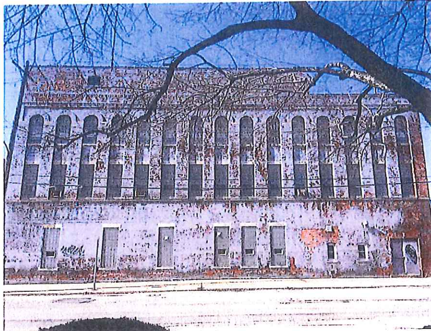
Photo 4: 445-449 10 th St. in 2018. North elevation. Credit: Erin Claussen
