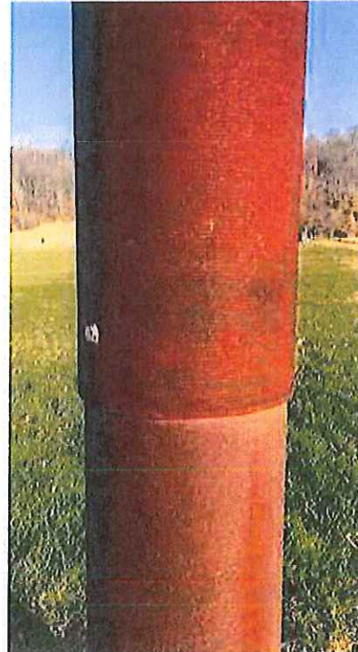
▶ Coated Finish Arc-applied zinc base coat with gray acrylic top coat
