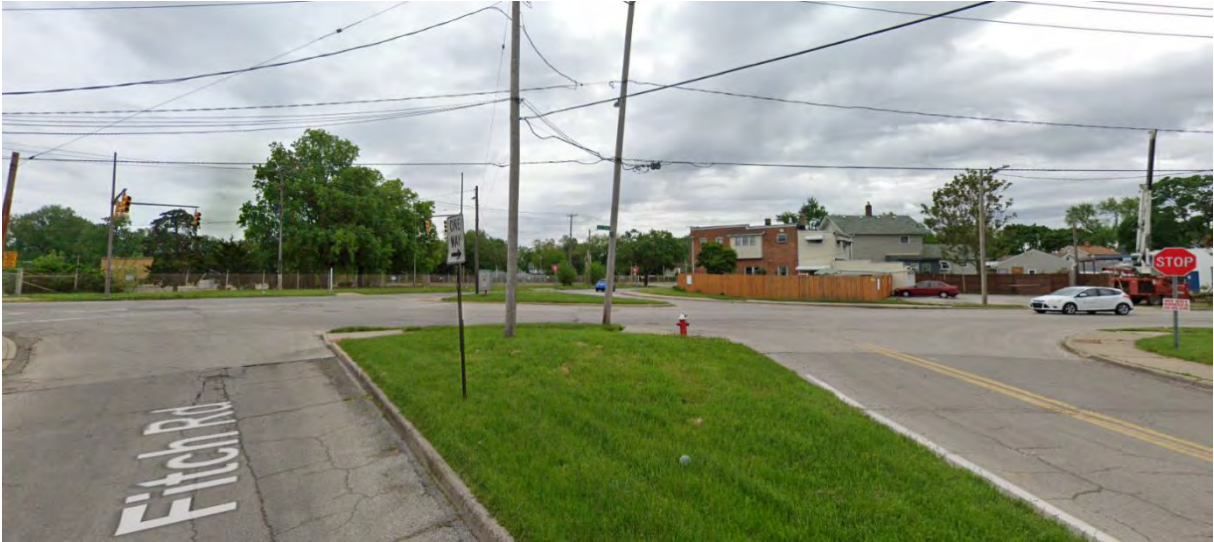
Figure 10 Missing crosswalk at the intersection of Fitch Road and Tremainsville Road
