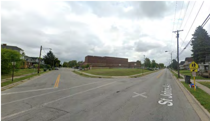
Figure 27 Wide curb radius at the intersection of Franklin Street and St Johns Avenue near South Science and Technology School
