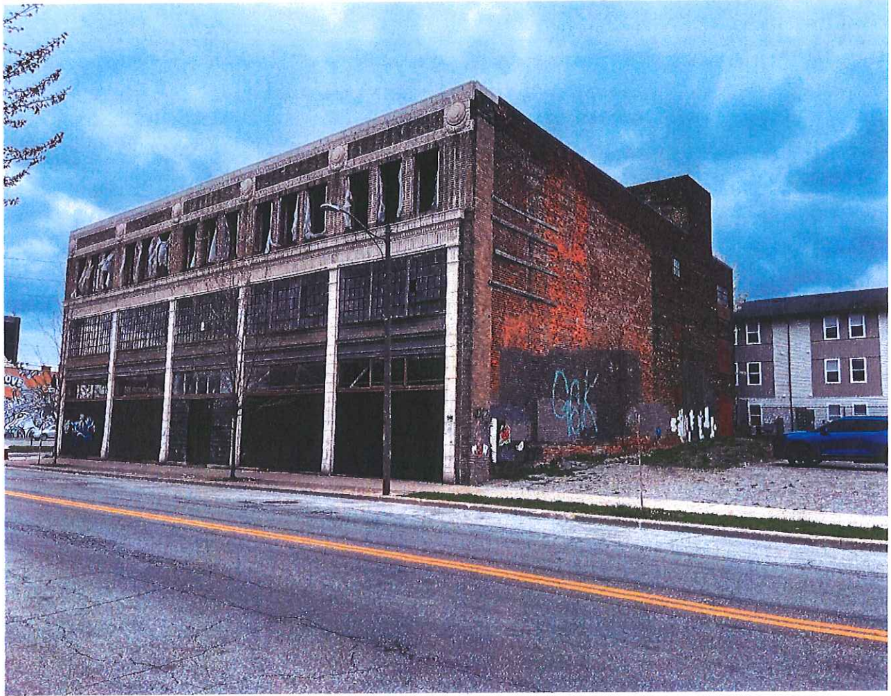
Plate 3: Looking south at main and northwest facades of 1301 Adams Street.
