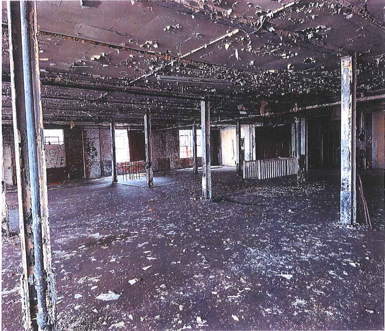
Plate 11: Second floor, looking northwest towards stairwell and rear facade
