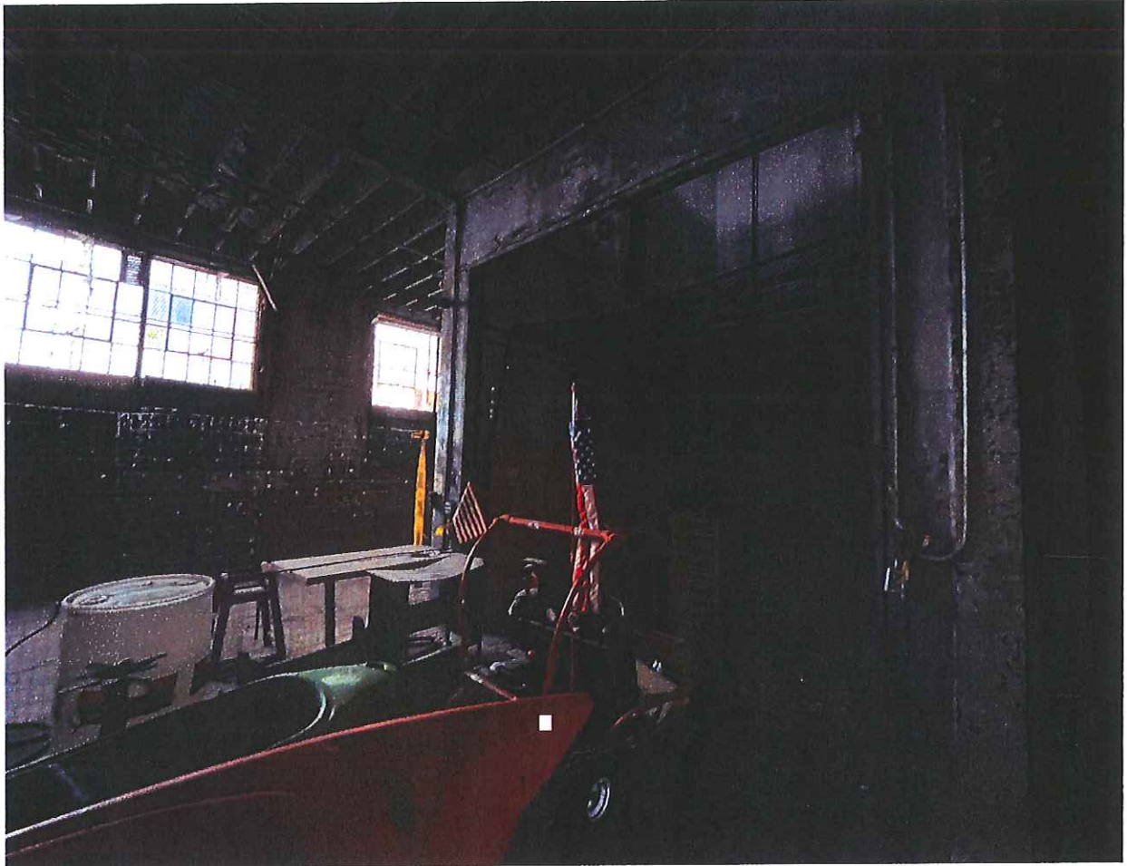
Plate 8: First floor rear garage/storage space, looking north-northwest toward Freight elevator.
