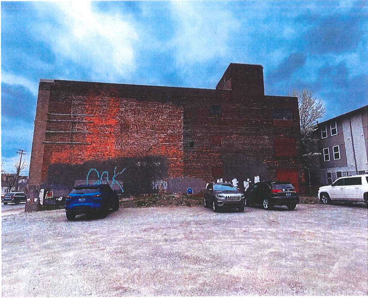
Plate 4: Looking east toward northwest façade of 1301 Adams Street.
