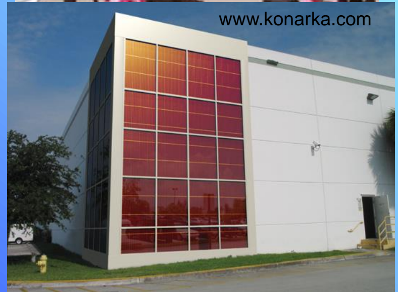
Solar "Curtain Wall"
