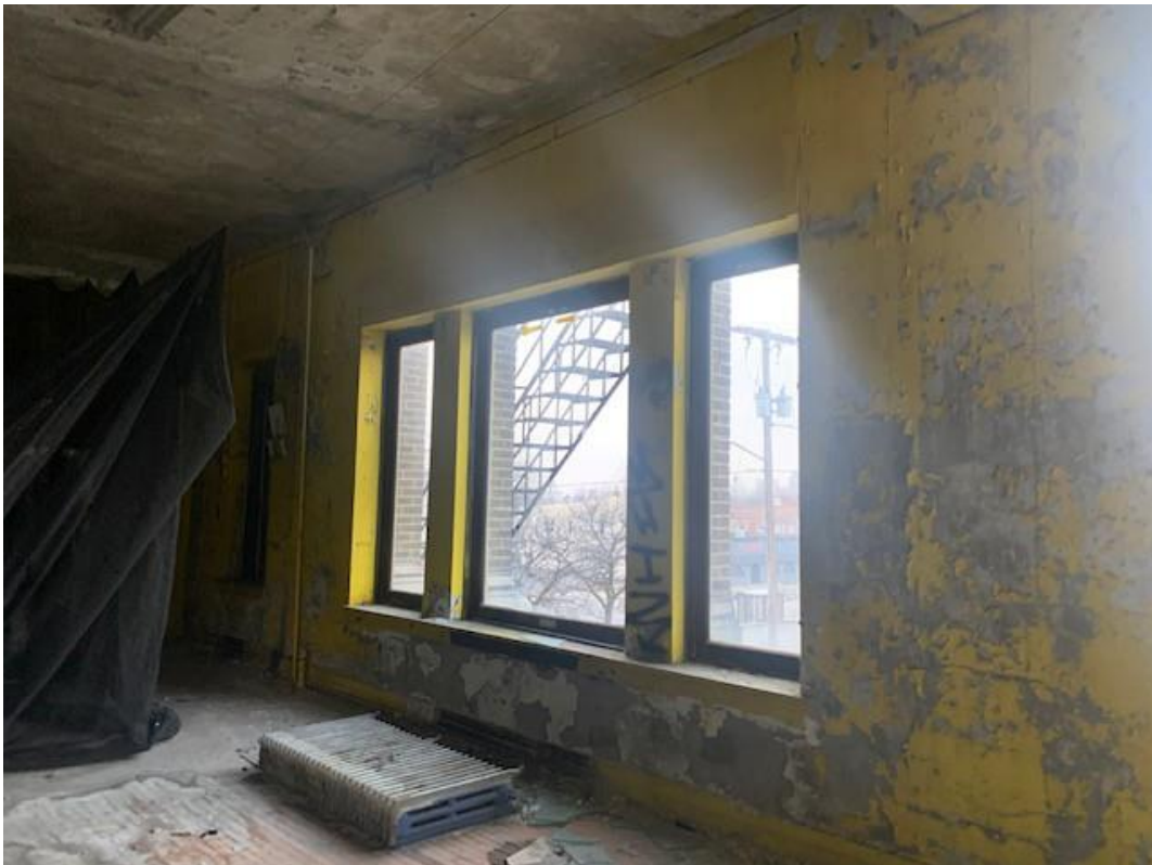
Photo 7: 401 S. Main St. circa 2020. Interior wall & window. Credit: ARK Development
