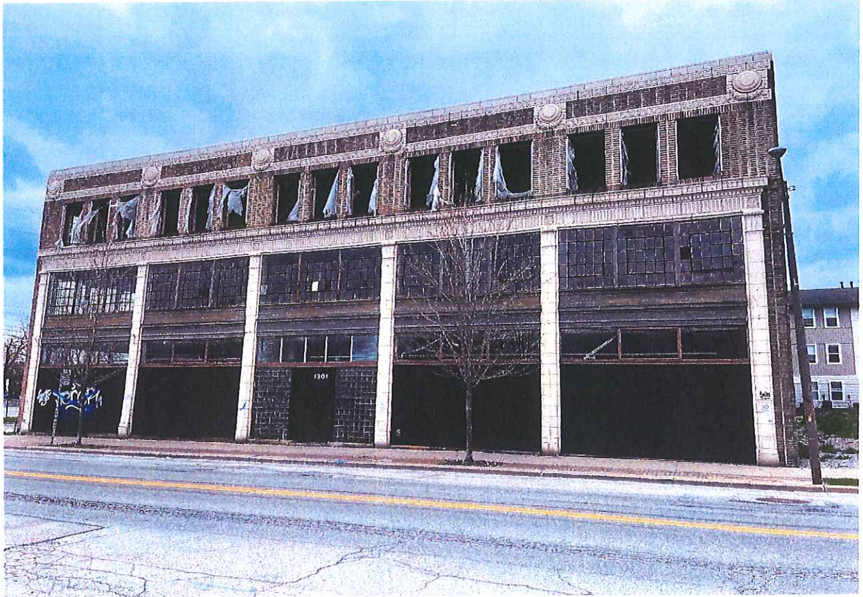
Plate 2: Looking southwest at the front façade of 1301 Adams Street.
