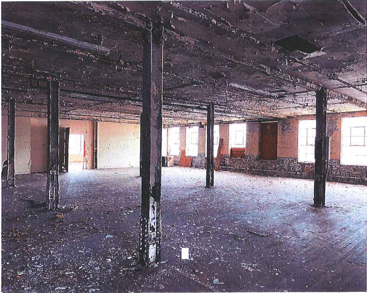
Plate 10: Second Floor, looking southeast towards 13 th Street, showing partitioned office space.
