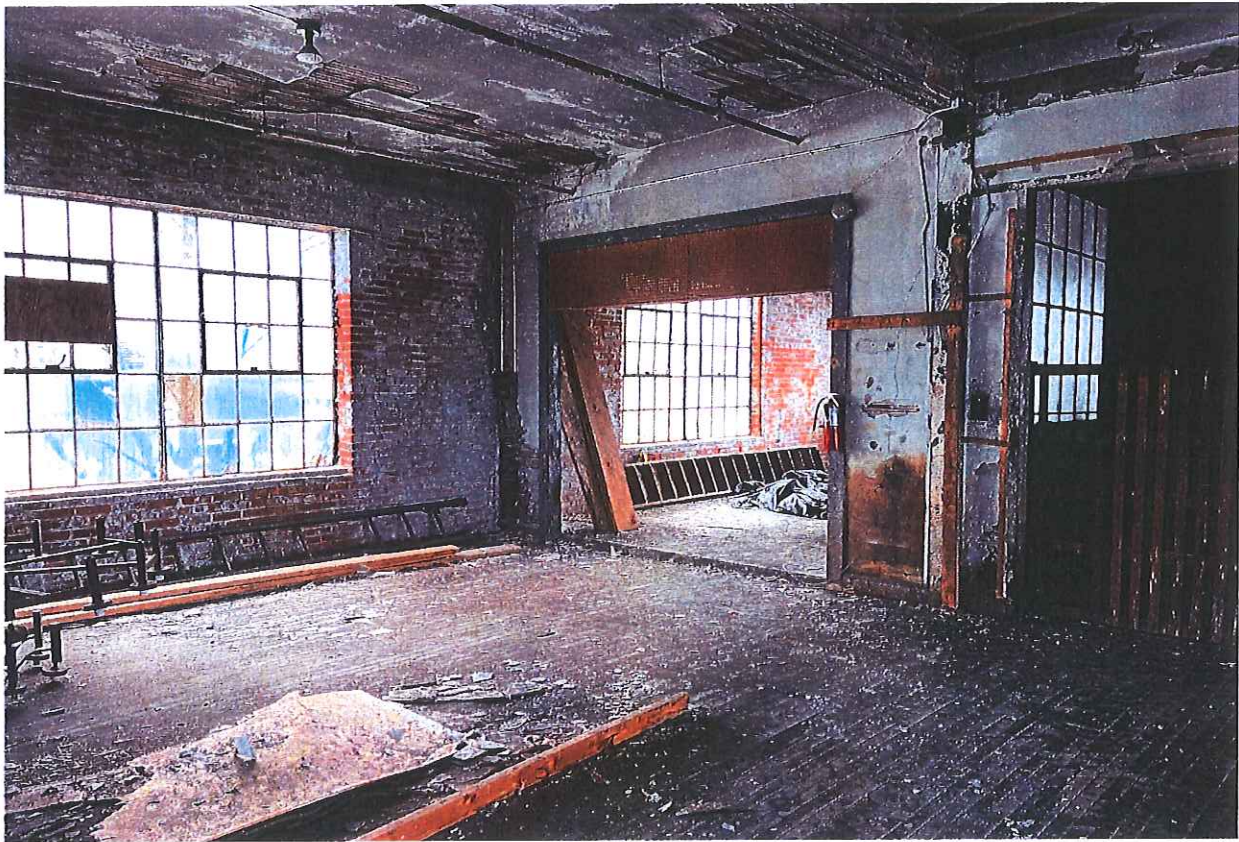
Plate 14: Third floor looking northwest toward freight elevator shaft and rear wall.
