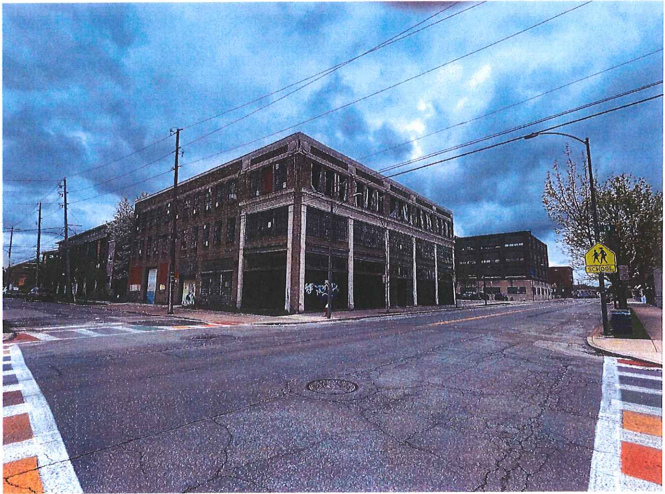
Plate 1: Looking northwest at 1301 Adams Street from Adams and 13 th Streets.
