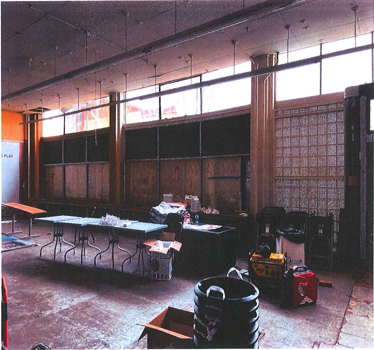
Plate 6: First Floor interior, looking northeast towards Adams Street façade.
