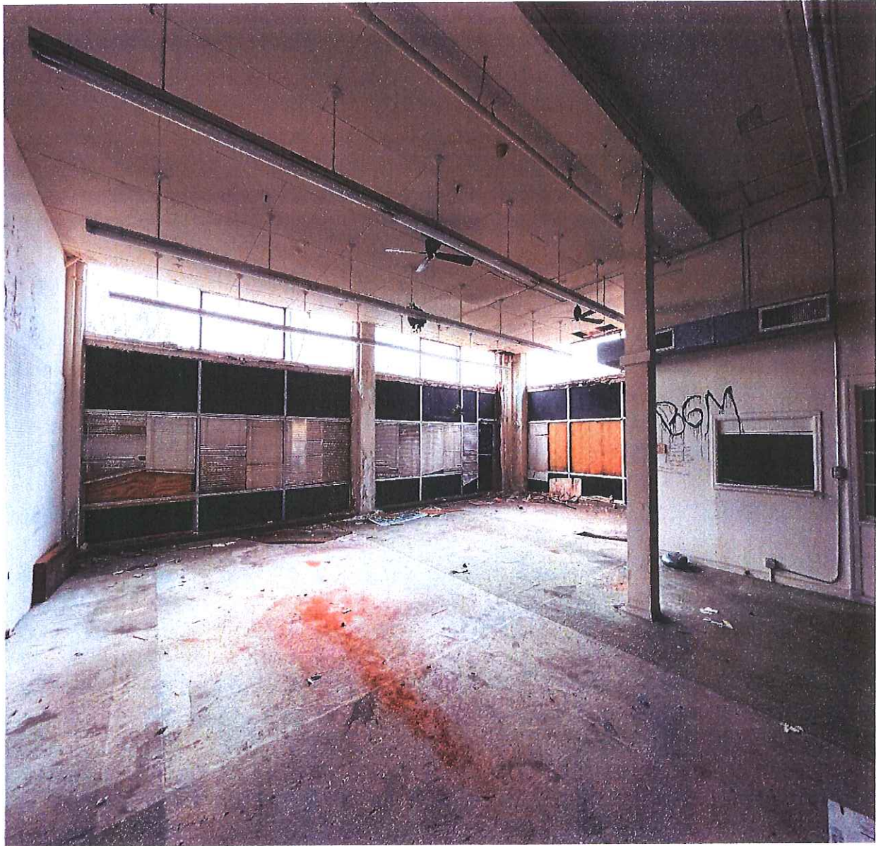
Plate 7: First floor, looking southeast towards Adams and 13 th Street corner.
